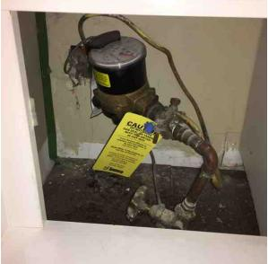
10.3.3 The water main pipe is only partially visible and suspected galvanized steel. A qualified plumber should further assess and upgrade / replace as required for improved water pressure / flow throughout the house and to prevent water damage due to corrosion-related water leakage.
